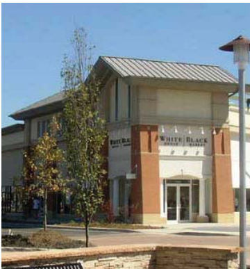
Commercial building with emphasis on corner treatment
