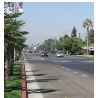
West El Monte Way looking west
